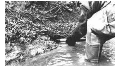
Dig pocket at water line.
